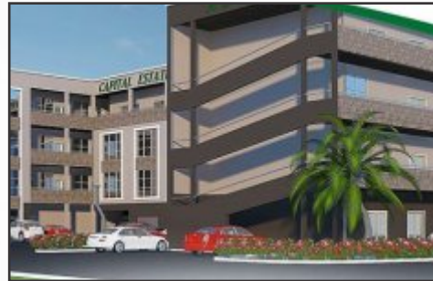
APDC Shopping Complex Units
